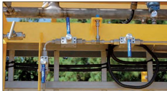
RIGHT: *The FKB series medium-pressure ball valve installed on the chemical injection skid.*
