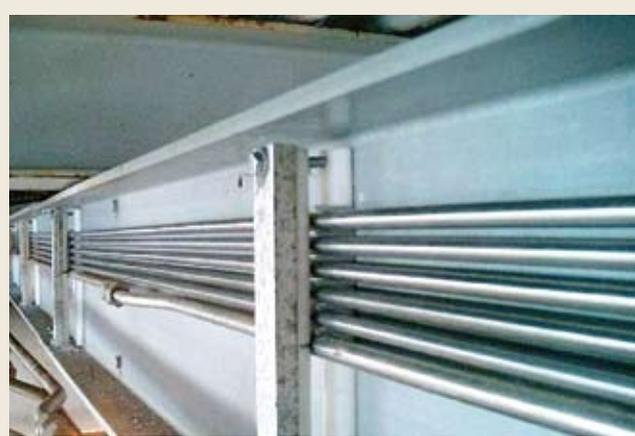
**Fig. 6.** Installation using 2507 superduplex tubing in the Gulf of Mexico. These tubing supports are based on half-round thermoplastic support rods.
